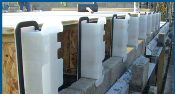
Plastic joist seals are another option for reducing air leakage associated with built timber joists. Courtesy of Manthorpe Building Products Ltd.
